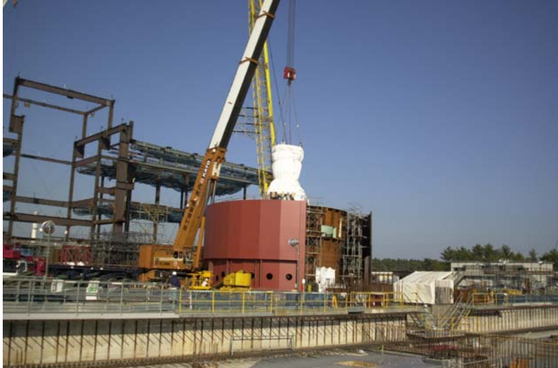
2004/12/03: Helium vessel was mounted above the helium vessel support cylinder.
