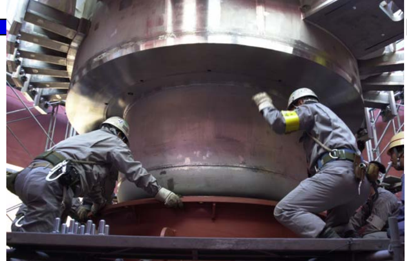
2004/12/03: Helium vessel was mounted above the helium vessel support cylinder.
