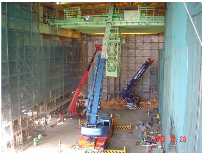
2005/10/28: 7.5t access crane was installed in the No.2 experimental hall.
