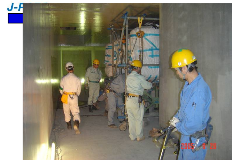
2005/09/26: Decay tanks for primary cooling system were installed in the basement.
