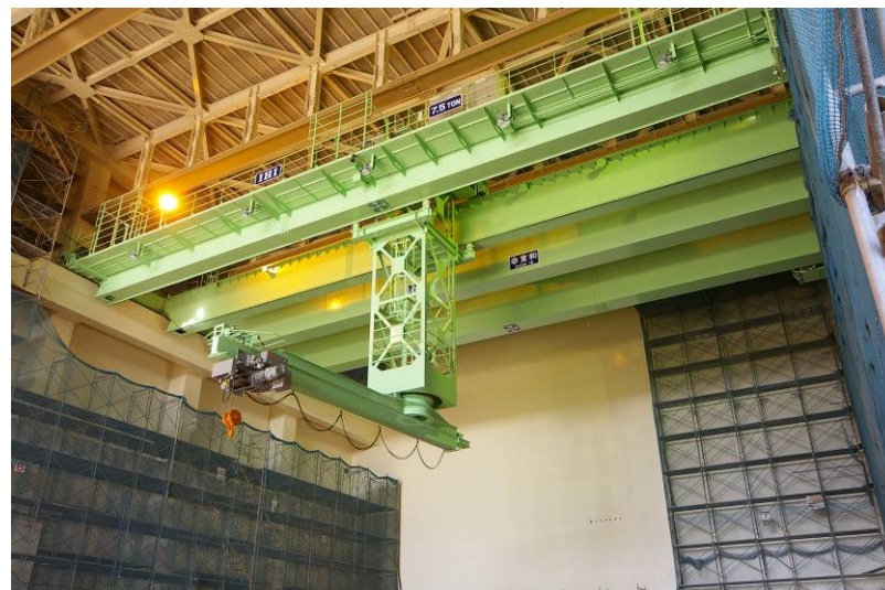
2005/11/04: 7.5t access crane was installed in the No.1 experimental hall.
