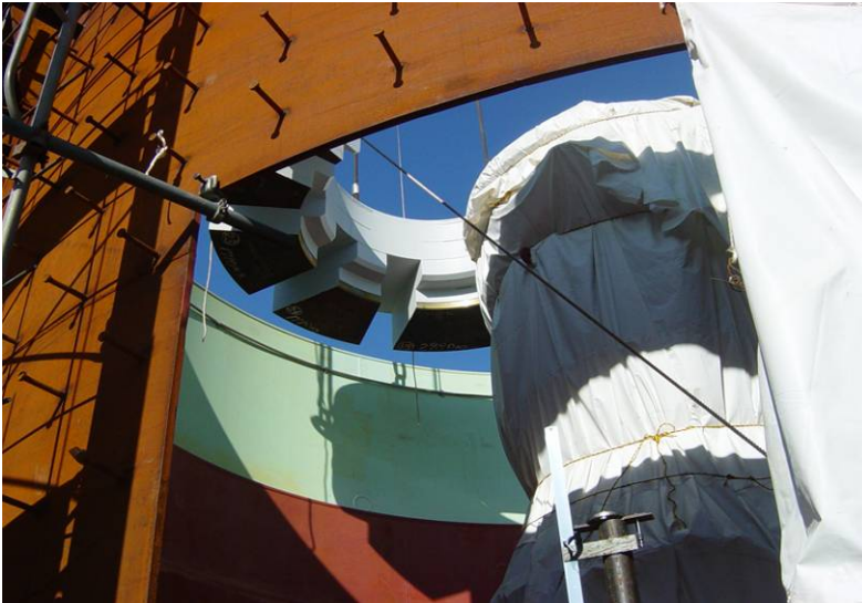
2004/12/17: Shielding blocks were mounted between the helium vessel and the outer liner.
