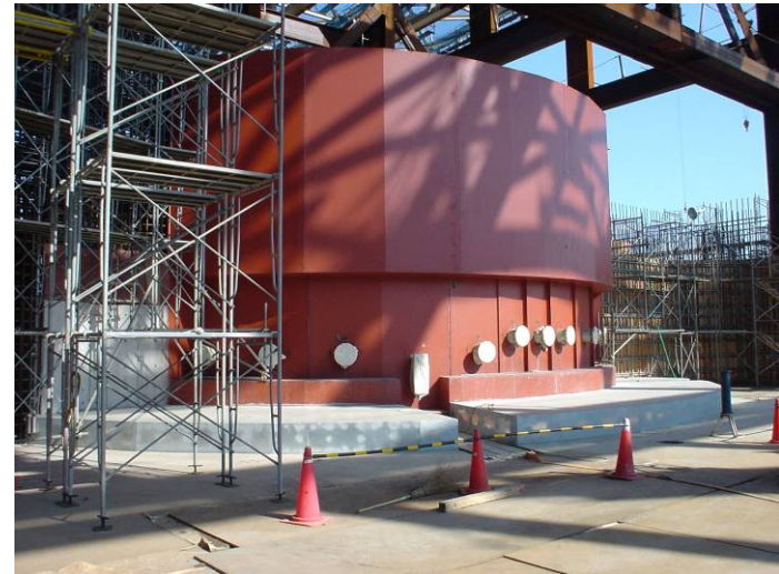
2005/04/01: Neutron Beam Port with concrete stage for pre-shielding blocks (West)
